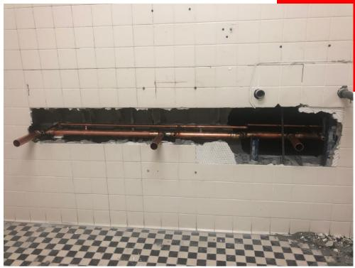
New Plumbing Piping installed for new Lavatories in 8<sup>th</sup> Street Building
